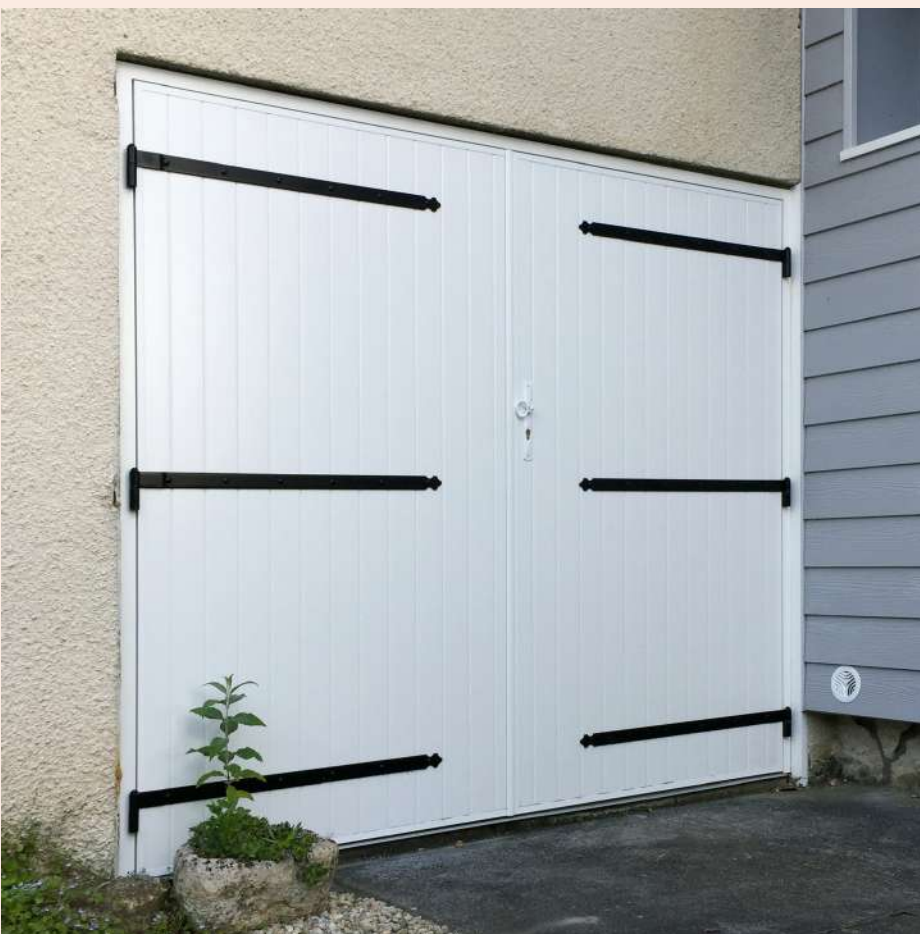
Panneau sandwich R = 0.28 \text{ m}^2.\text{K}/\text{W}
